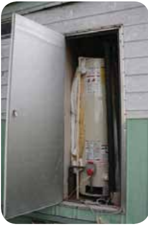
Water Heater Cabinet
