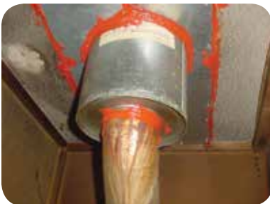
Sealing a flue with metal flashing and high temp caulk
