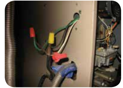
Improper gas & electric connections
