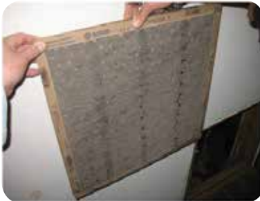
Replacing a dirty furnace filter
