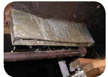
Combustion air inlet
