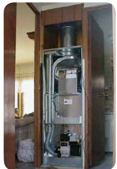
New Sealed Combustion Furnace
