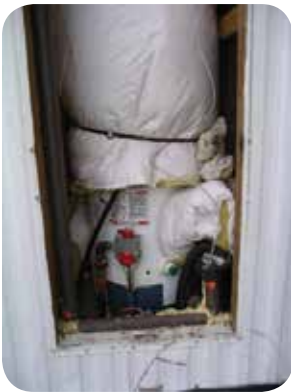
Air sealing and tank insulation
