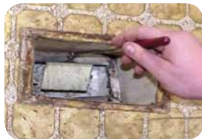
Duct inspection with mirror
