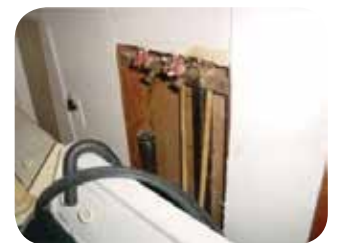
Open wall cavity after plumbing repair.
