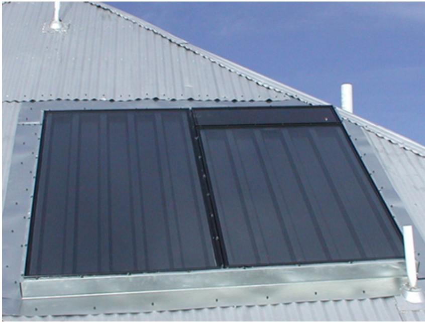
Flat-Plate Air Collector on a barn roof.
